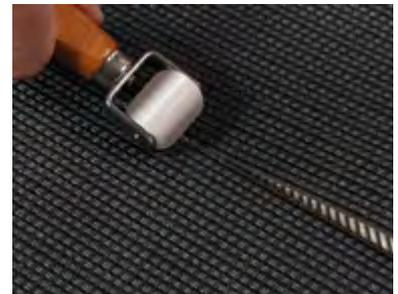
**8.** Refold the strips, carefully joining the two edges for a smooth seam and ensure the seal with the seam roller; then smooth out the entire area with the heavy roller to remove any air bubbles.
