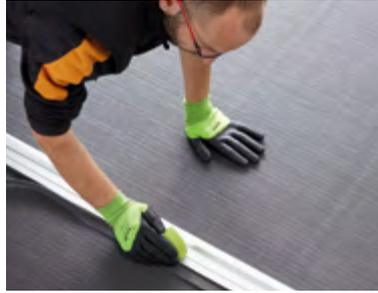
**2.** Using a ruler and Stanley knife or other adapted tools (railcut of Wolf, tiptop of Janser...), proceed with the double cut. Cut through both thicknesses at once, in the middle of the two strips' overlap. Remove remnants and check the seam's quality. If the cut is not perfect, renew the operation.
