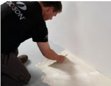
**6.** Uniformly apply the glue to the first half of the strip using a grooved spatula, but without allowing glue strands to form.
