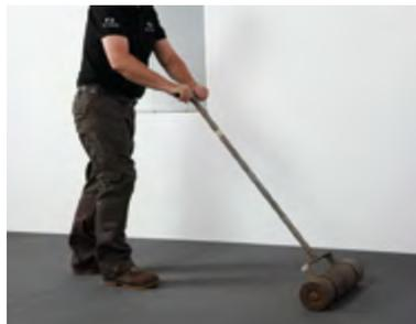
**10.** Press firmly into place, working out any air bubbles with the smoothing roller. Fold up the other side of the strip and repeat steps 6, 7, 8 and 9.
