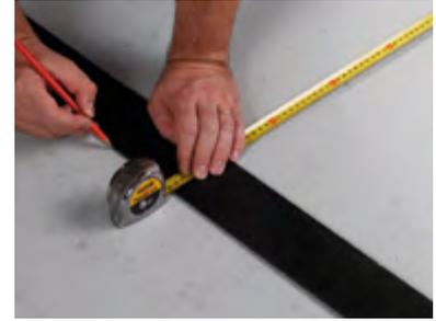
**3.** Mark the exact position of the initial strip while making sure to leave enough room in both directions for the levelling.
